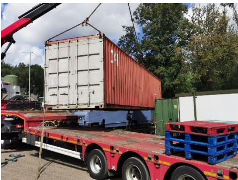
Lowering the new container into place
